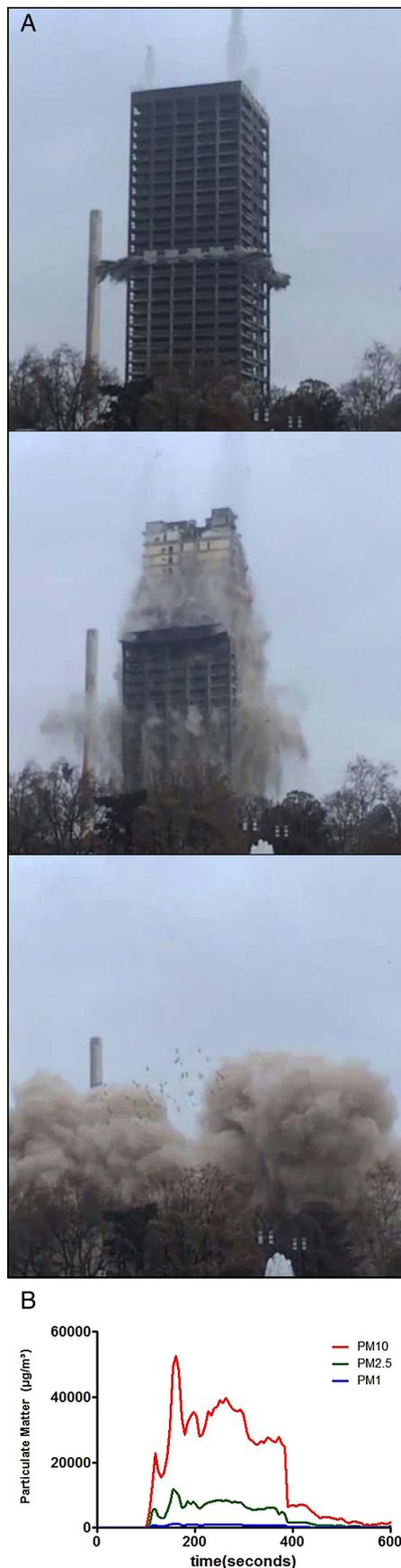
**Figure 1** (A) Three pictures of the detonating AFE Tower in Frankfurt am Main, 2 February 2014. (B) The graph documents the concentration of PM<sub>10</sub>, PM<sub>2.5</sub> and PM<sub>1</sub> in  $\mu\text{g}/\text{m}^3$  for several minutes during the collapse of the building. PM, particulate matter.
